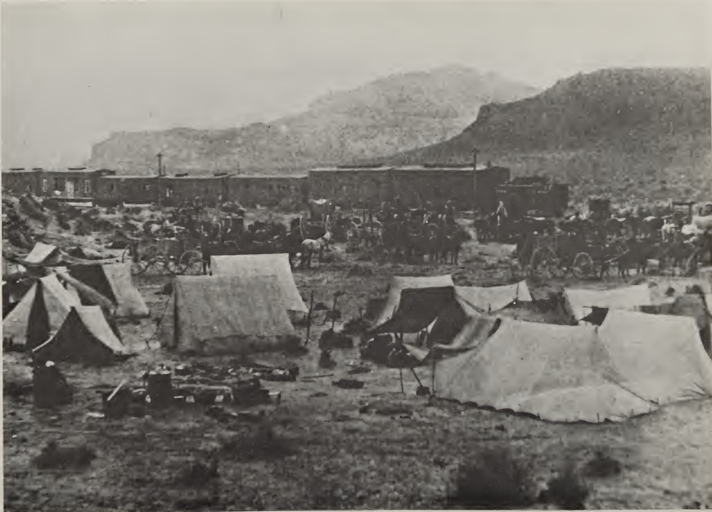
Figure 7: Railroad construction camp (Southern Pacific, Alfred A. Hart Photograph).
